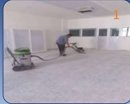
PREPARATION DE SUPPORT
